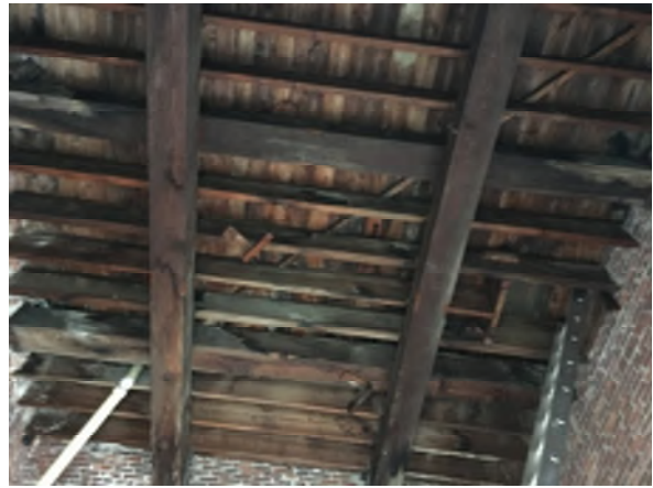
BELL TOWER FLOOR FRAMING
