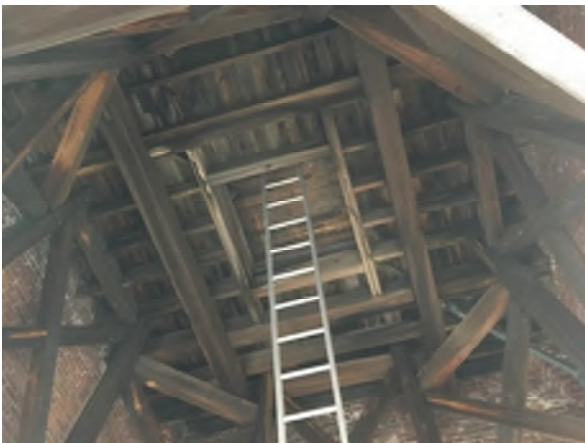
BELL TOWER ROOF FRAMING
