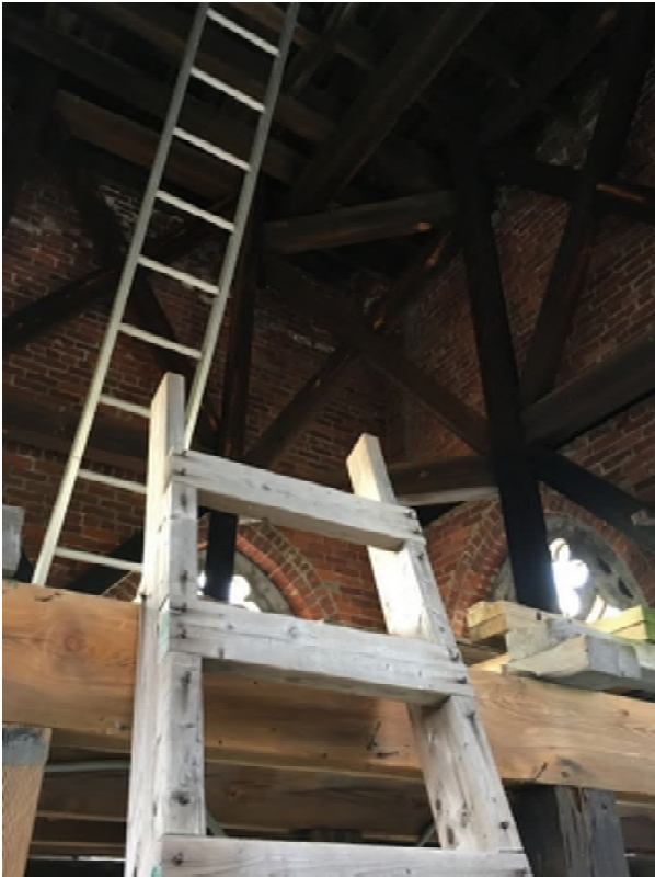
BELL TOWER TIMBER BRACING
