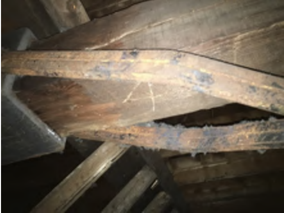
STEEL RODS MAIN ROOF TRUSS NEAR DETAIL A
